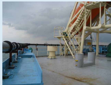
Installed Bondstrand on the aft deck
