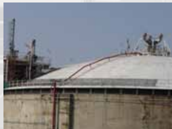
Riser pipe to central spreading unit (T-302)
